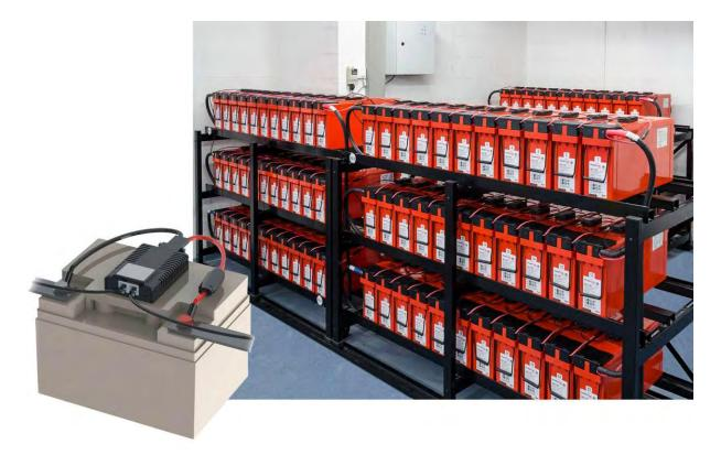
GENEREX's 3<sup>rd</sup> generation BACS<sup>®</sup> (**B**attery **A**nalysis & **C**are **S**ystem) is the most advanced product of its kind on the market today. An ethernet integrated battery monitoring and management system, BACS<sup>®</sup> uses web management technology to monitor the temperature, internal resistance, and voltage of every single battery in a given system.
